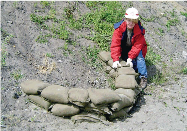
Corps employees demonstrate building a ring dike.
