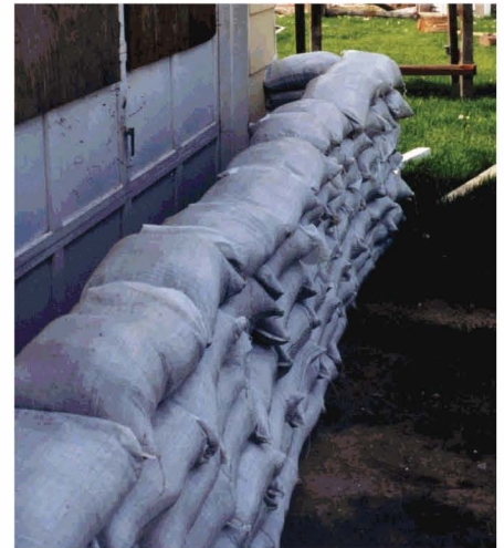
Single stack placement
