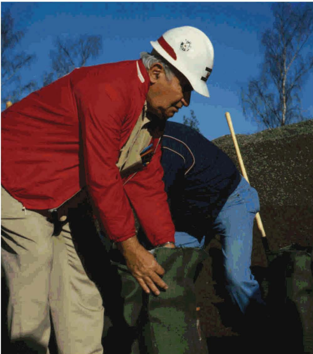
Veteran flood engineer Ernie Sabo demonstrates that the sandbag should be two-thirds full, folded at the top.
